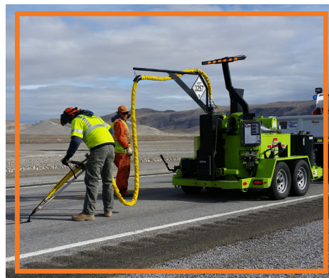
Crack Sealing
